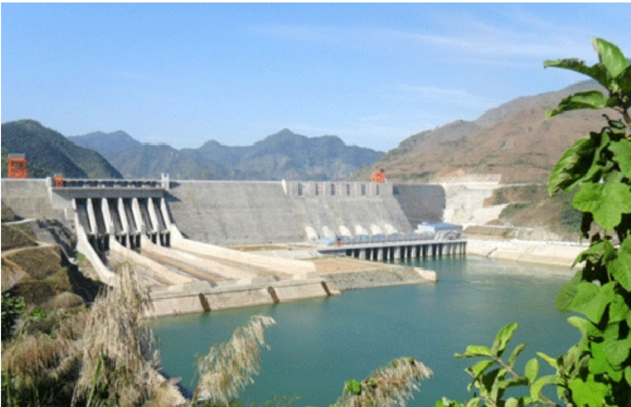
Figure 17 – Son La Hydropower Plant - a renewable energy source for the Ta Khoa Project
