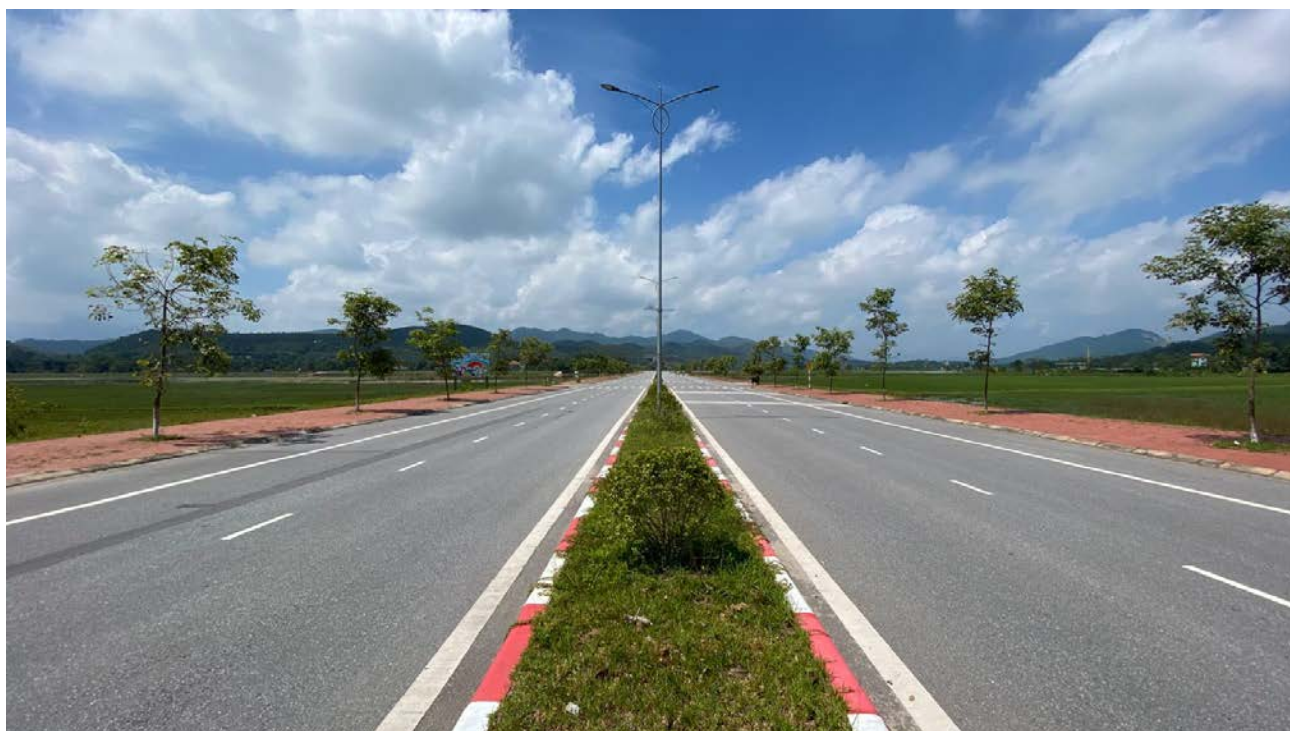
Figure 19 - Highway 37 - sealed road to the Ta Khoa Project
